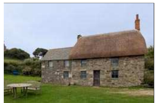
Thatched Roof House near Prussia Cove
